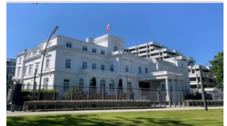
Hamburg Former Consulate
